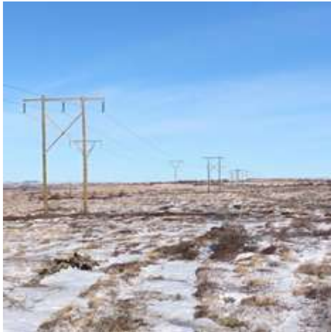
Figure 14: Repairs Complete on TL219
